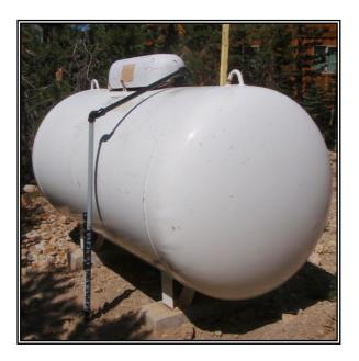
systems to accomplish this. The first is a precast reinforced concrete pad that sits under the tank legs.
