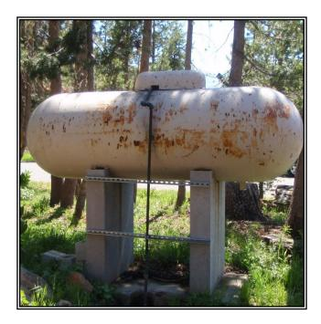
The second system uses saddles, which are precast reinforced concrete devices that allow a tank to sit off the ground. Saddles can be a few inches to a maximum of four feet tall at the belly of the tank. They have a round cutout shape that corresponds to the configuration
